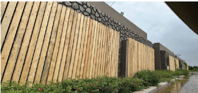
Wooden planks installed to prevent damage to glass barriers
